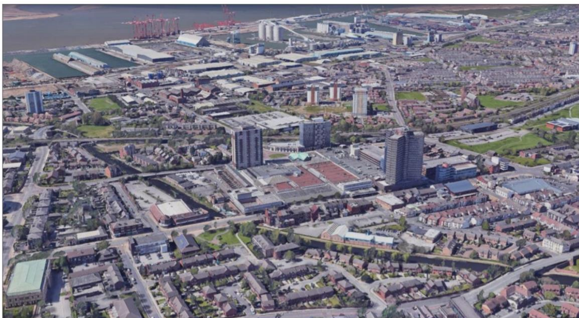
Figure 7 Bootle Town Centre, including the Strand Shopping Centre, viewed from the south east towards the River Mersey
